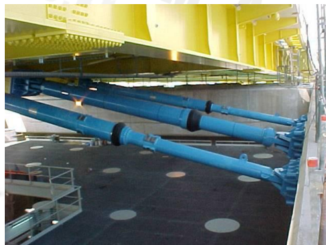
5) Earthquake damper
